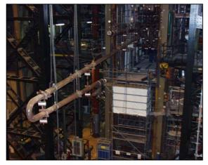
Phenix : disassembling of a SG module for repair
